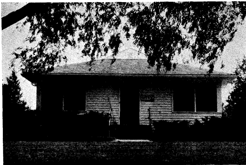
Fig. 18.—The new office building constructed in 1948 at a cost of $12,920. "It is located across the main drive from the superintendent's residence."
