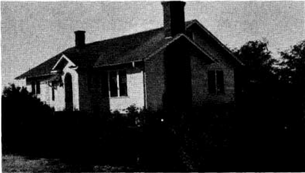
Fig. 16.—The superintendent's cottage after it was remodeled in 1932.
