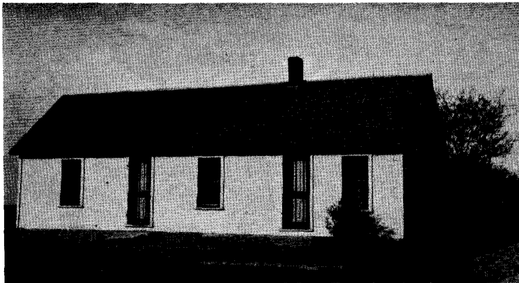
Fig.14-- "The first office building constructed from the smaller of the two granaries purchased with the farm. The building, 16 by 40 feet, was placed on a concrete foundation and divided into three sections--an office, a laboratory, and an exhibit room."
