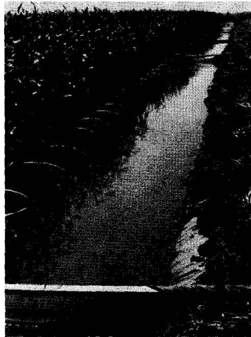
Fig. 21.-Head ditch on irrigation project. "Fields are irrigated with gated pipe where possible. Other fields were irrigated by the open-ditch-siphon-tube method."
